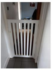
A gate was required to limit access to a kitchen for a young boy. The gate is a wooden construction that is dowelled and glued together. As always the difficult part was establishing a locking mechanism which prevented Logan from opening the gate. In discussion with the client it was agreed that the gate would be key locked. A door security bolt with rack bolt key was used. The key was stored on
