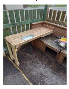
As can be seen the extension was at 90 degrees to the existing Mud Kitchen with the worktop raised to allow wheelchair access under it. The worktop was made from treated wood planks screwed together with stainless screws and corner brackets. Support blocks (with spacers to ensure a level worktop) were screwed to the existing Mud Kitchen walls to provide a positive location for the worktop. A rectangular stainless steel trough was provided to give better access.
