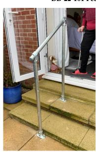
Lady, difficulty walking, lives in bungalow, wants handrail to be able to exit bedroom by patio doors and descend 3 steps to the garden. Patio doors open from centre outwards, so rail needs to be in centre of steps. A rail was constructed from 42mm galvanised rail with bases bolted down to the patio slabs.
