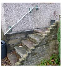
The client has dementia and needed a hand rail fitting to garden steps which lead to "favourite" bench in the garden. Α rail attached to the side of the garage which flanks one side of the steps - see photo. The hand rail is made from standard 42.4 mm diameter galvanised
