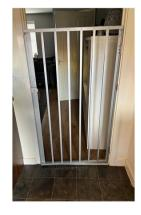
A young boy with complex needs required a safety gate to limit his free movement around his home. The gate was made to a previous design using aluminium extrusions pop riveted together. The gate was mounted using lift-off hinges so it could be removed when not needed to give better access.
